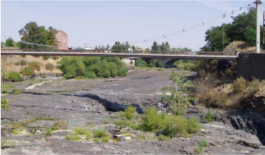
North Channel of Upper Falls without water.
